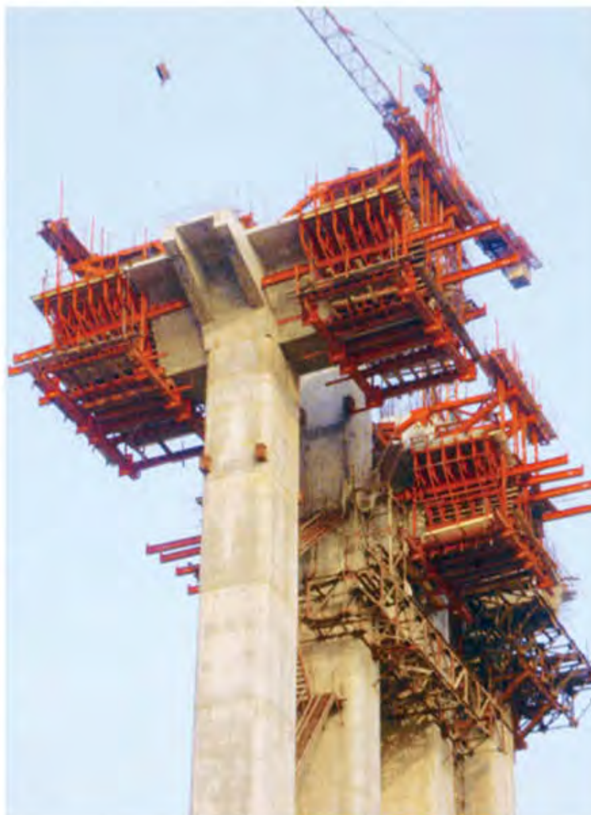
钢挂篮 HANGING BASKET CONSTRUCTION CRANE
