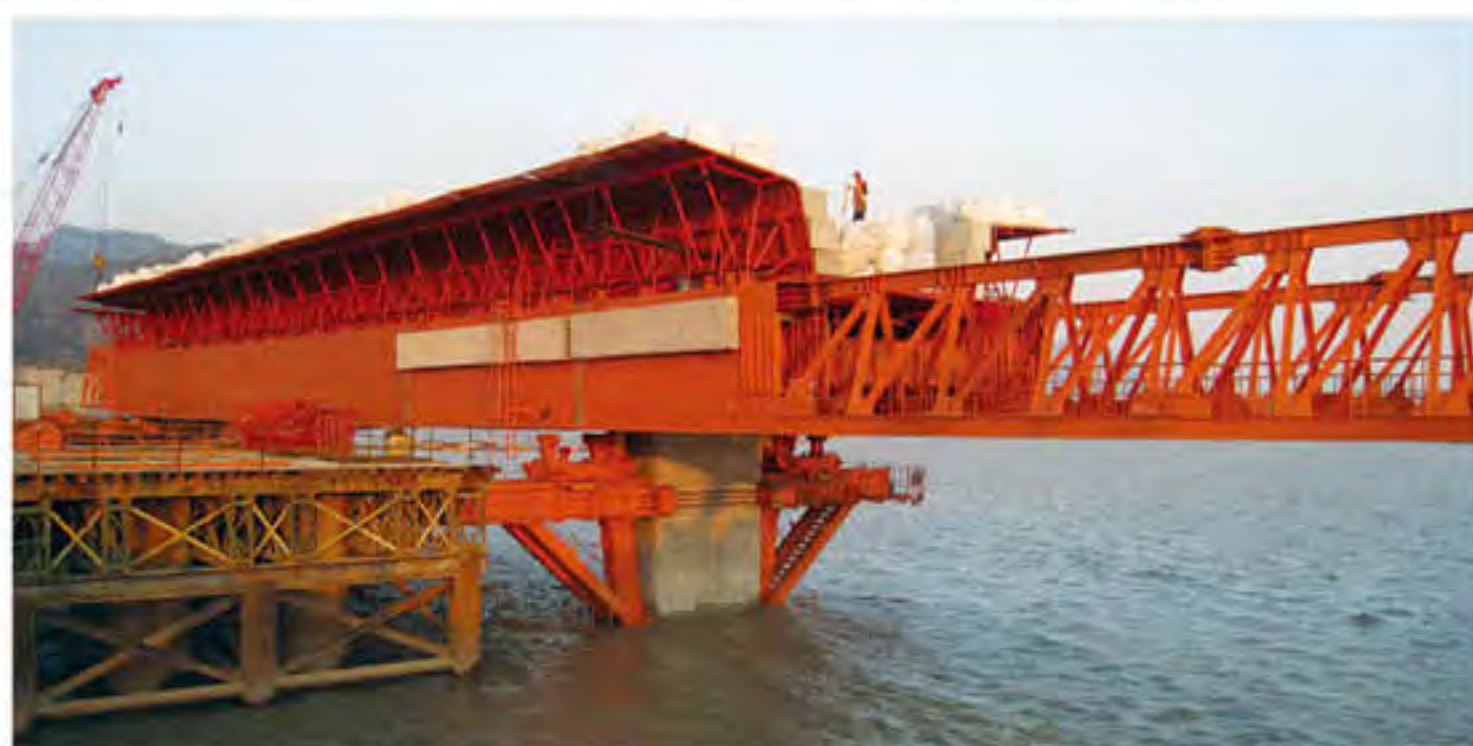
移动模架 BRIDGE ERECTING CRANE
